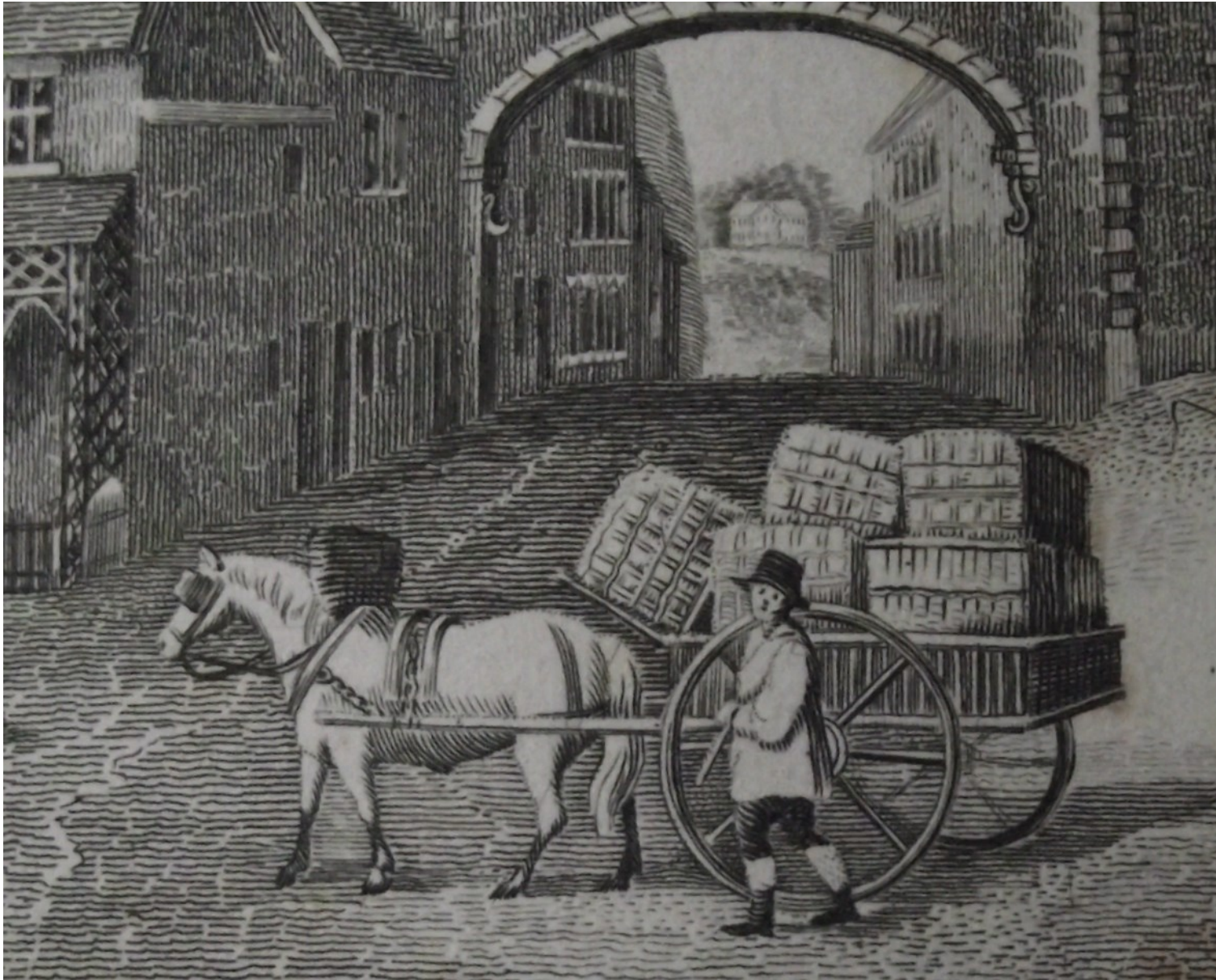
From John Ward's Borough of Stoke-upon-Trent , 1843. Detail of the East Front of the Manufactory of Enoch Wood & Sons, Burslem.
